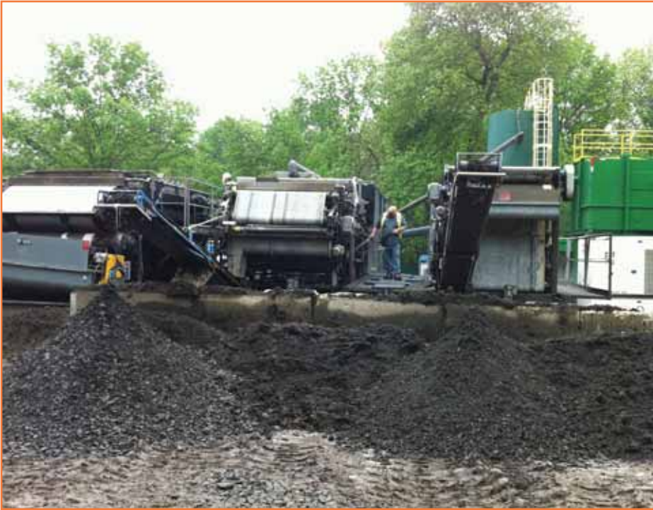
Dewatered silts, clays & organic sediment after being processed through JND's plant.
