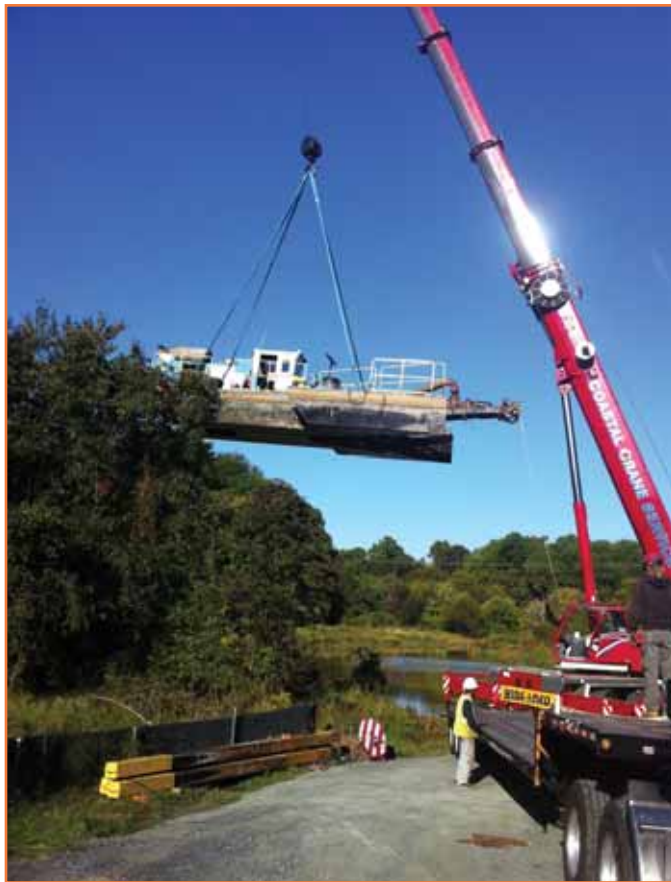
Unloading of Moray dredge at Wilde Lake.
