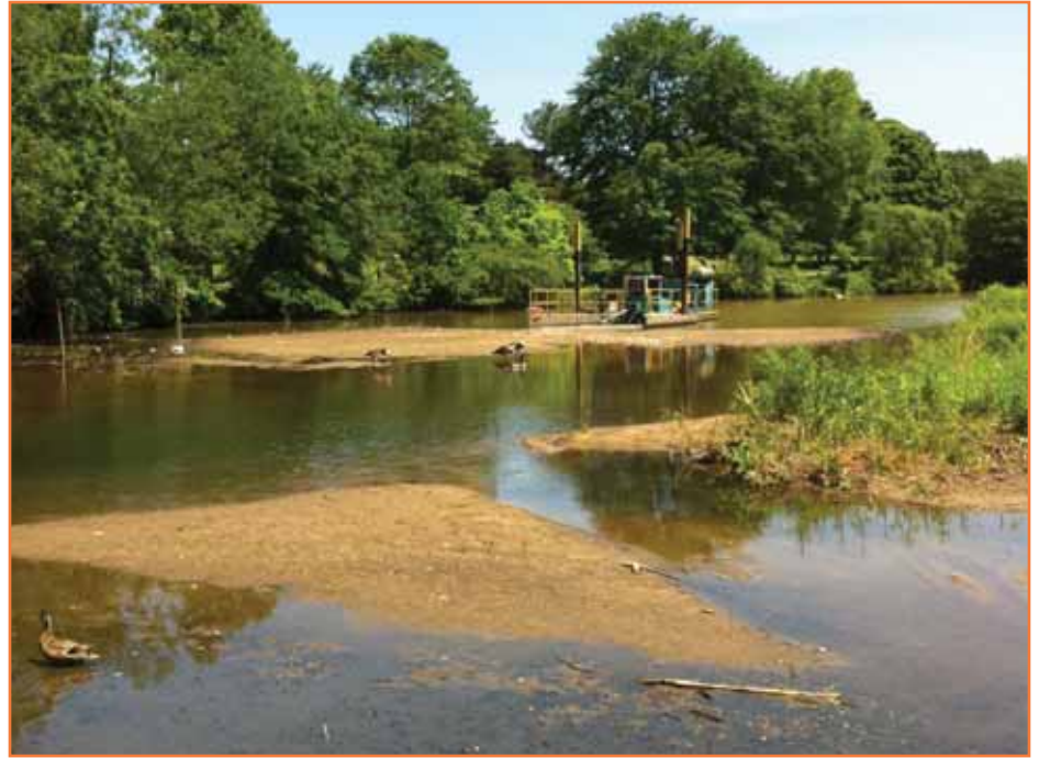
Dredge removing accumulated sediment at inlet of Wilde Lake.
